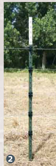
1. H brace for the start of a 5-wire fence. 2. T-Post along the line of a 5-wire fence. 3. Wood post along the line of a 5-wire fence.
