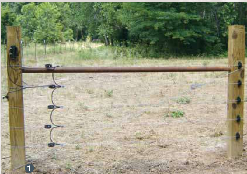
1. H brace for the start of a 5-wire fence. 2. T-Post along the line of a 5-wire fence. 3. Wood post along the line of a 5-wire fence.
